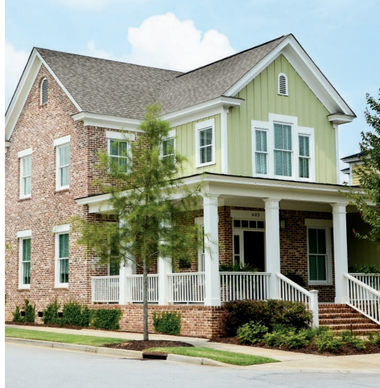
FEATURED ABOVE // LEGEND DOUBLE HUNG WINDOWS FEATURING 5-1/2" FLAT CASING WITH BULL NOSE SILL NOSING MANUFACTURED WITHOUT HEAD CASING. CUSTOM HEADER APPLIED IN THE FIELD. North Augusta, South Carolina.
